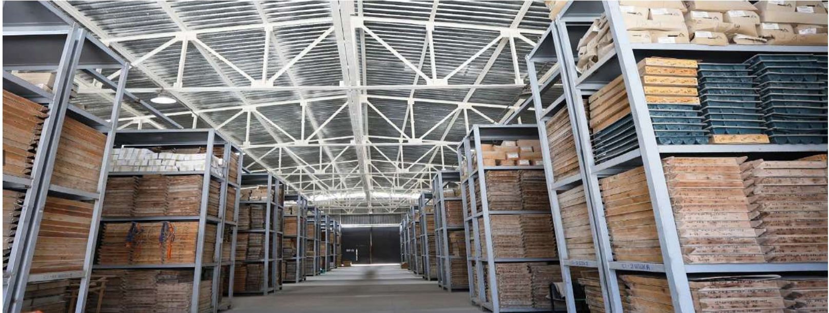
One of the AMMC core storage warehouses — a capacity of 60,000 boxes
