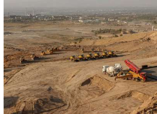
Construction of the Yoshlik-I open pit and CEP-3
